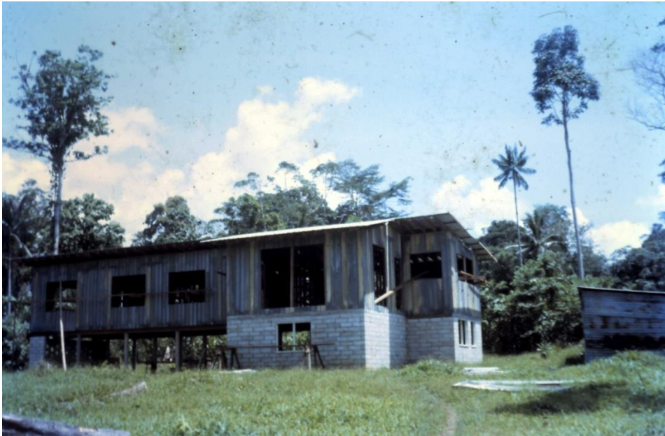
Principal's home under construction.
