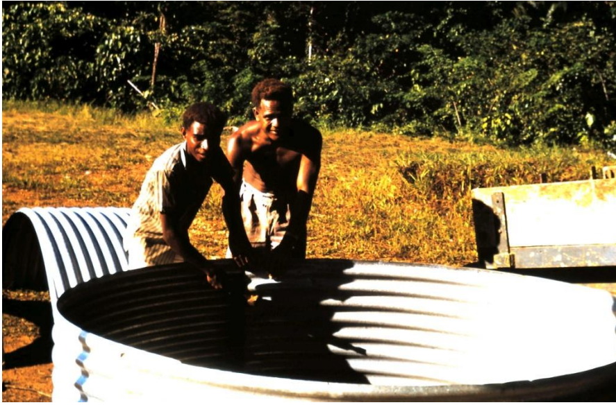
Anga and a student assembling a water tank for the school.
