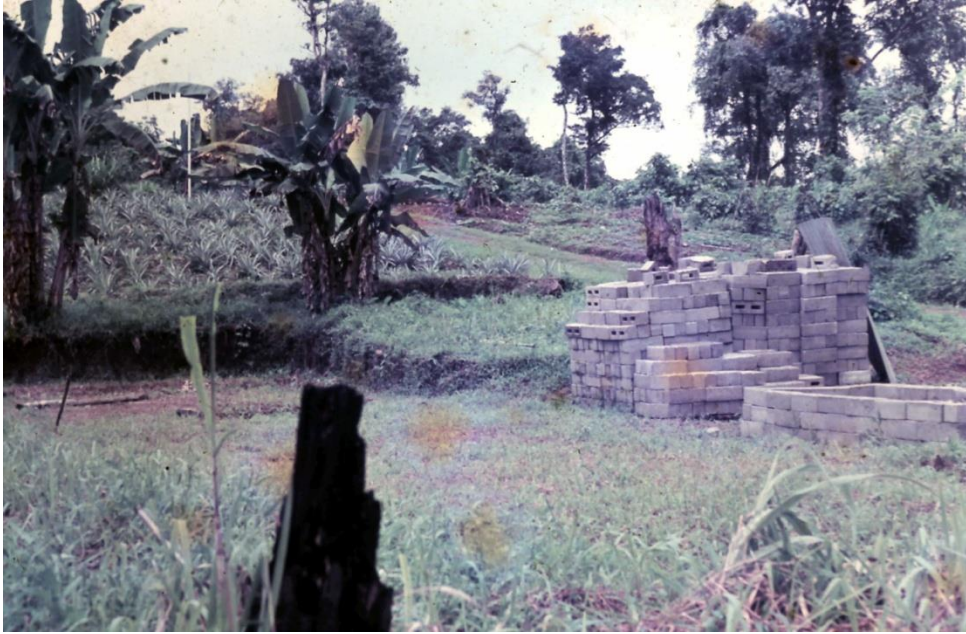
Concrete Blocks made from the Limestone ready for the new Girls' Dorm. Note the Pineapples and Bananas growing on the slope behind the site.
